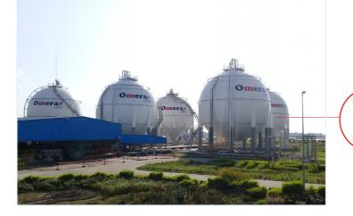
3 EPC for the construction of 4 LPG storage and bottling plants with two spheres of 2,200T each, in Mongla / Dhaka / Bogra / Chittagong. Construction of a LPG river barge of 300T.
