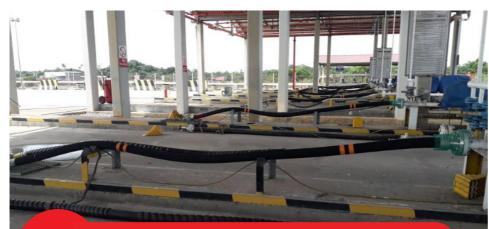
ELAFLEX LPG hoses installed at Quantum LPG Terminal – Atuabo. The remaining LPG Bulk Distribution Depots i.e. Tema Fuel Company, Blue Ocean and Matrix also have ELAFLEX LPG hoses installed for LPG Loading Constant supply of ELAFLEX ZVA Nozzles and Safety Breakways to major service companies like Universal Engineering, Rich Morgan, and GPS Tokheim for use at TOTAL, SHELL, GOIL and other OMCs Fuel Dispensing Stations
